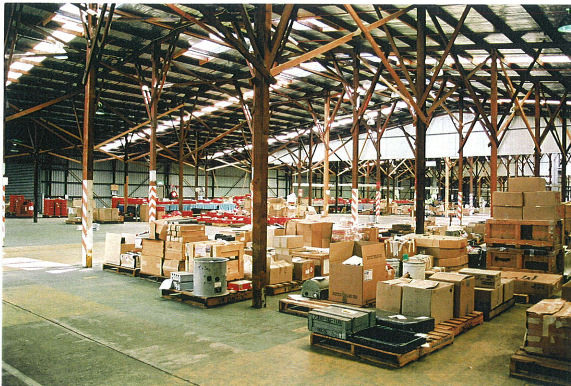
Fig. 3.3 TYPICAL INTERIOR OF A WORLD WAR II TIMBER POST AND BEAM STORE BUILDING AT DNSDC MOOREBANK
