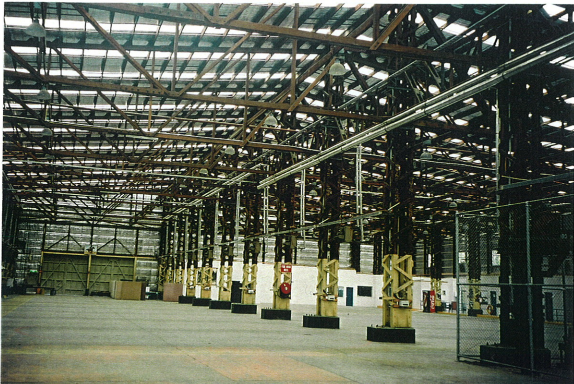
Fig. 3.6 INTERIOR WORKSHOP 105, REFURBISHED FOR USE BY THE ARMY RESERVES, SHOWING TIMBER CONSTRUCTION
