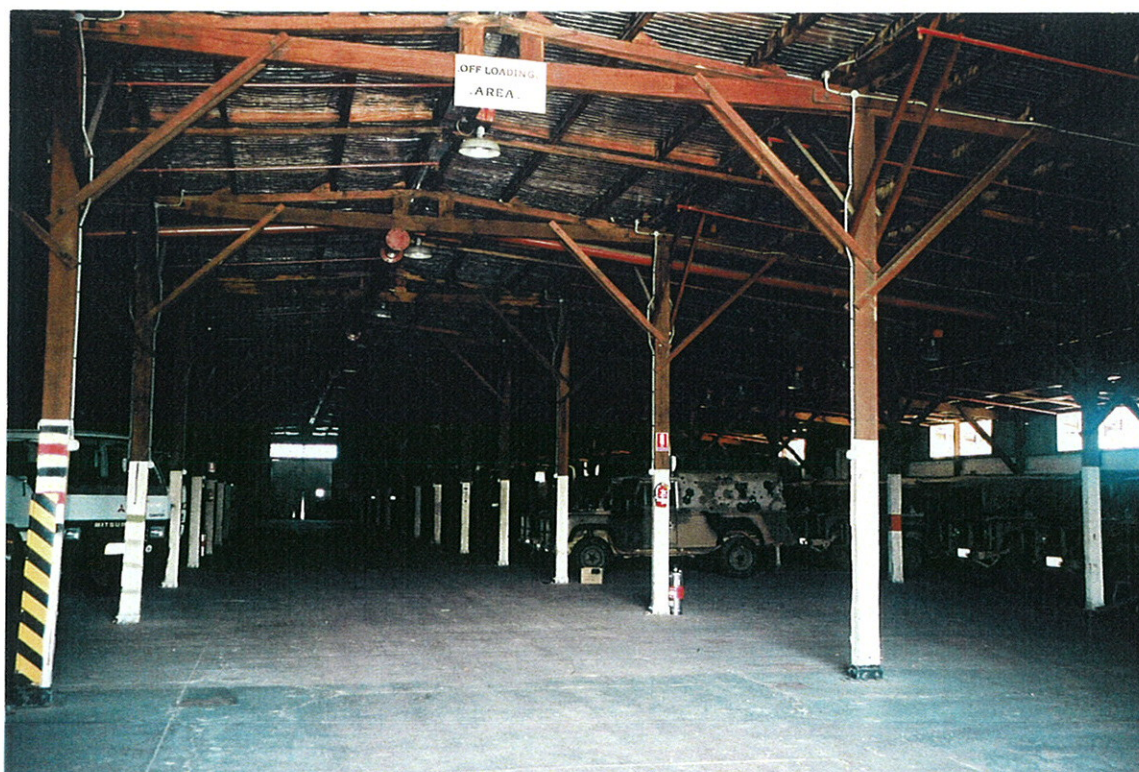
Fig. 3.8 INTERIOR OF A TYPICAL TIMBER POSTS AND BEAM STOREHOUSE AT NORTH BANDIANA, SHOWING SIMILAR TIMBER CONSTRUCTION TO THAT FOUND AT DNSDC
