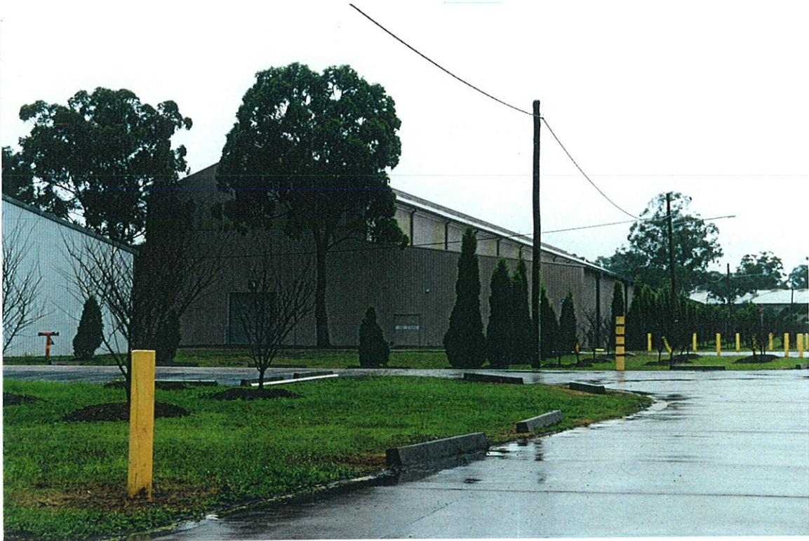
Fig. 3.1 BUILDING 9 AT THE CENTRE OF THE DNSDC SITE, A TYPICAL WORLD WAR II COMPOSITE TIMBER AND STEEL WAREHOUSE BUILDING, OF WHICH THERE ARE THREE AT THE SITE, AND WHICH HAS BEEN REFURBISHED DURING THE EARLY 1990s.
