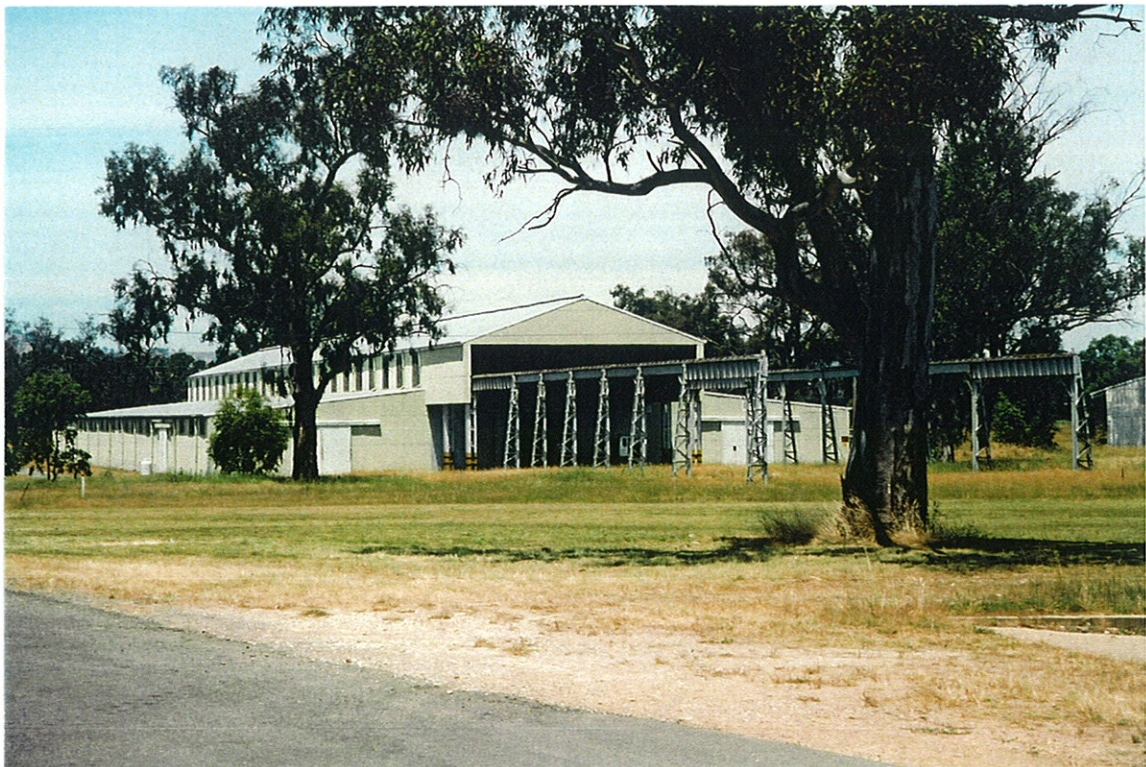
Fig. 3.10 ONE OF THE THREE TRANSIT STORES AT NORTH BANDIANA, WHICH HAVE A COMPOSITE TIMBER AND STEEL CONSTRUCTION SIMILAR TO THAT FOUND AT DNSDC
