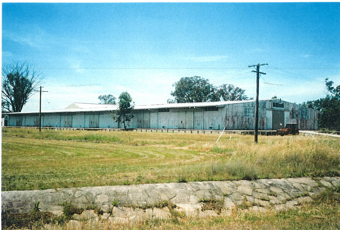
Fig. 3.7 TYPICAL EXAMPLE OF THE EIGHT TIMBER POST AND BEAM STOREHOUSES CONSTRUCTED ON CONCRETE PLINTHS, LOCATED AT NORTH BANDIANA
